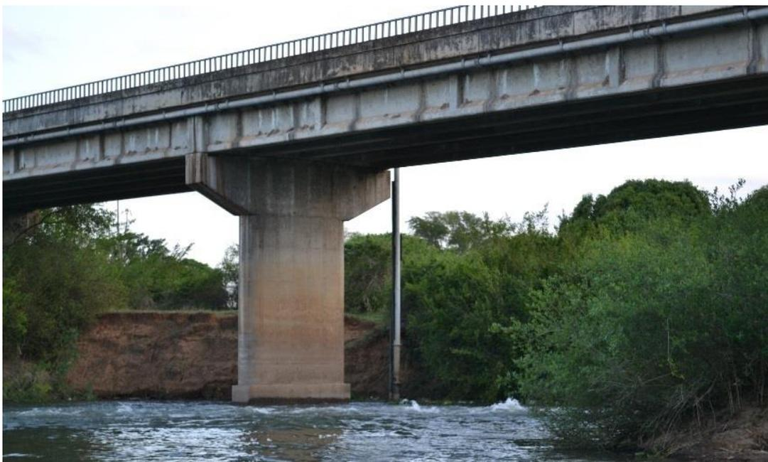
**Figure 9.10** Stage gauge W4H010 attached to bridge pier at Lake View (M. Kempen, undated).
