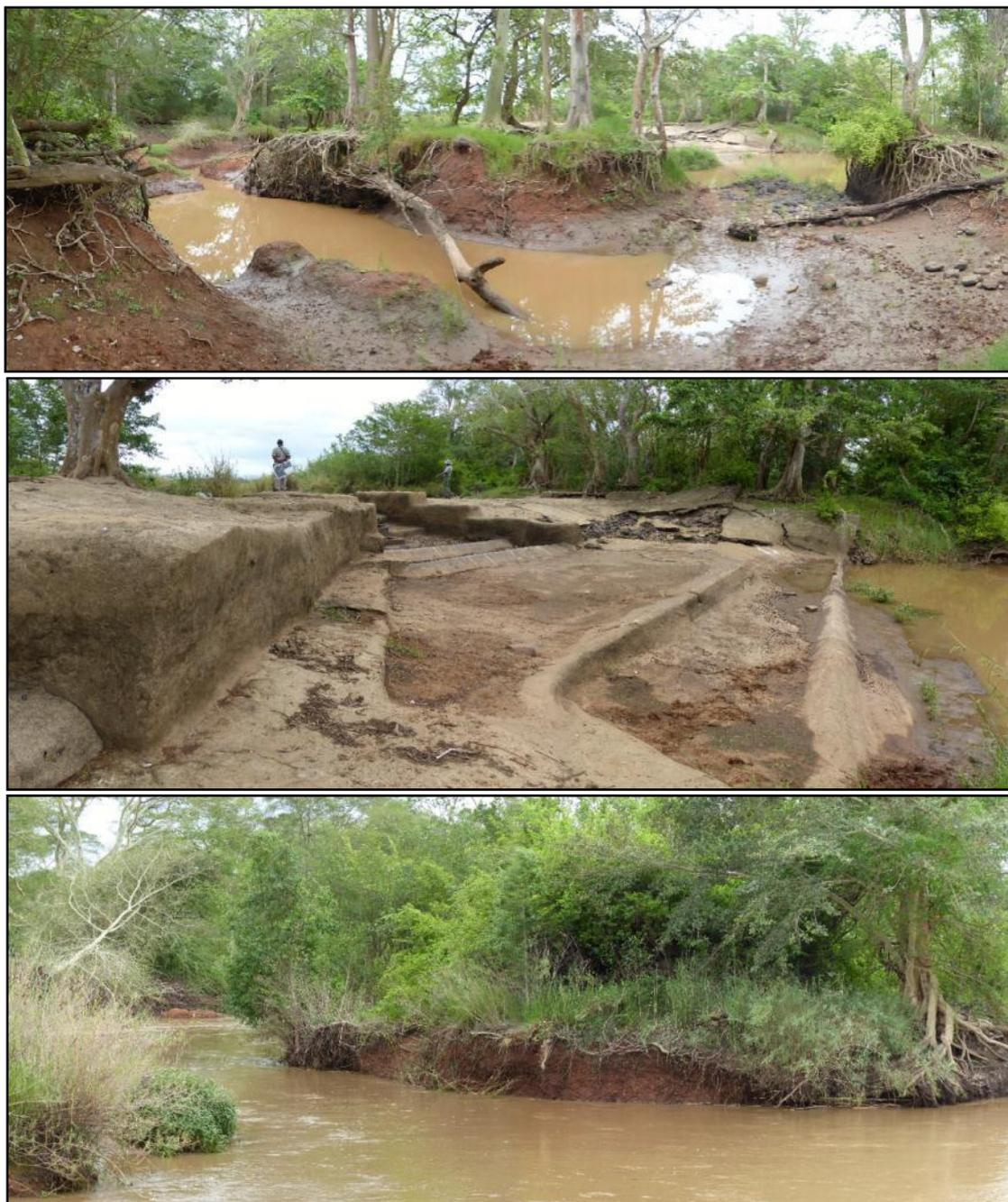
**Figure 4.3** Photographs of Banzi Pan showing: (top row) incision/channel in the *Ficus* forest resulting from elevated flows around the southern end of the weir; (second row) the weir at the historical pan outlet; and (bottom row) channel incision resulting from elevated flows (now the main channel) around the northern end of the weir (November 2014).
