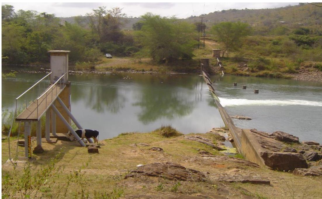
**Figure 9.9 Discharge gauging station W4H013 located downstream of the Jozini Dam Wall (refer to Figure 9.3; DWAf 2008).**
